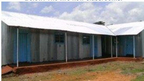
Below: The two new classrooms.
